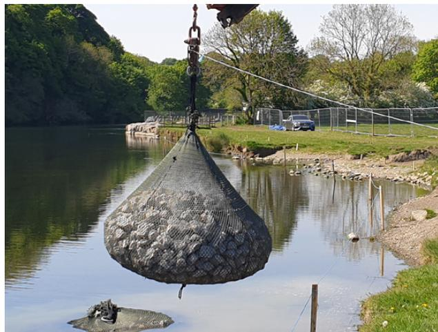
The AquaRockBag® is an environmentally friendly, highly durable net, which is filled with larger sorted stones and is used to protect against erosion and scouring, as well as in landscape (re)modeling.
